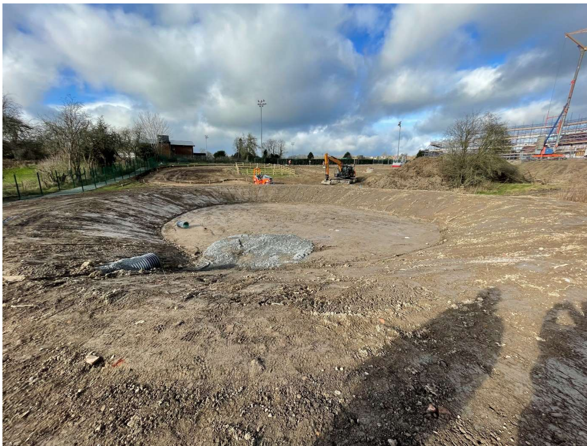
FIGURE 4.1: CONSTRUCTION OF A POND AT YSGOL GYMRAEG Y TRALLWNG IN 2022.
